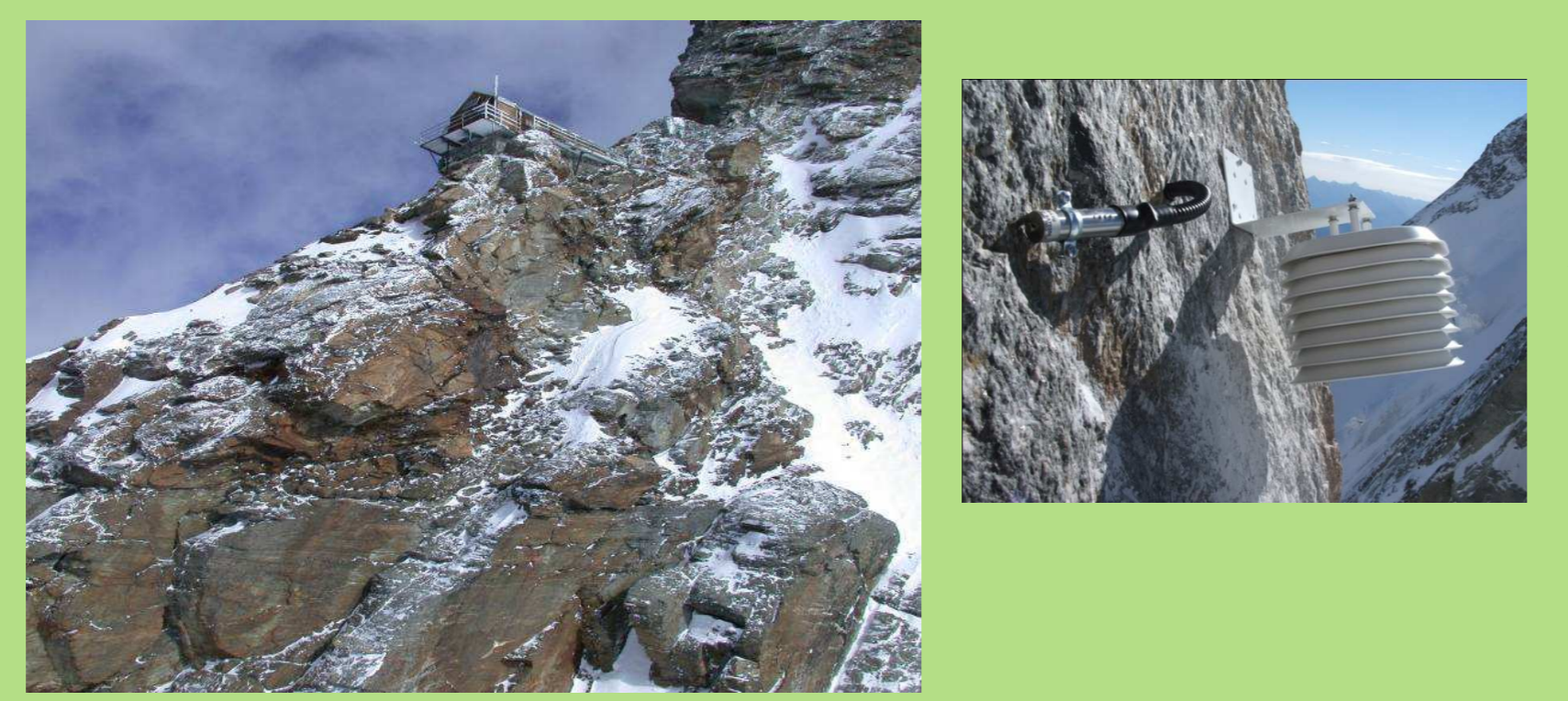
Fig1. Example of an high-mountain infrastructure affected by permafrost degradation (Carrel Hut – Matterhorn). The complex topography strongly affect rock thermal regime. In the small picture the mini-datalogger used for the monitoring of rock and air temperature.
